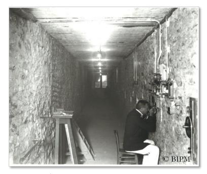
Charles-Édouard Guillaume measuring in the 24 m long geodetic base installed in the basement of the Observatory.
