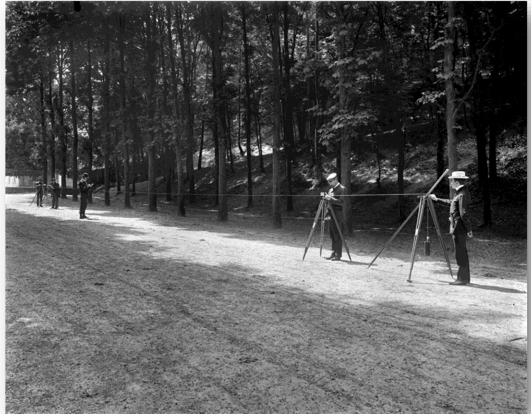
Guillaume carrying out measurements with invar threads and the improved Jäderin apparatus at the BIPM (© Jacques Boyer_Roger-Viollet)
