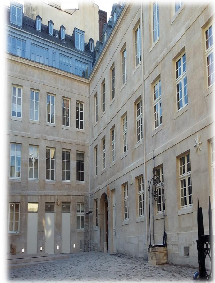
The new entry of the Bureau des longitudes at the Institut de France (© Martina Schiavon)
